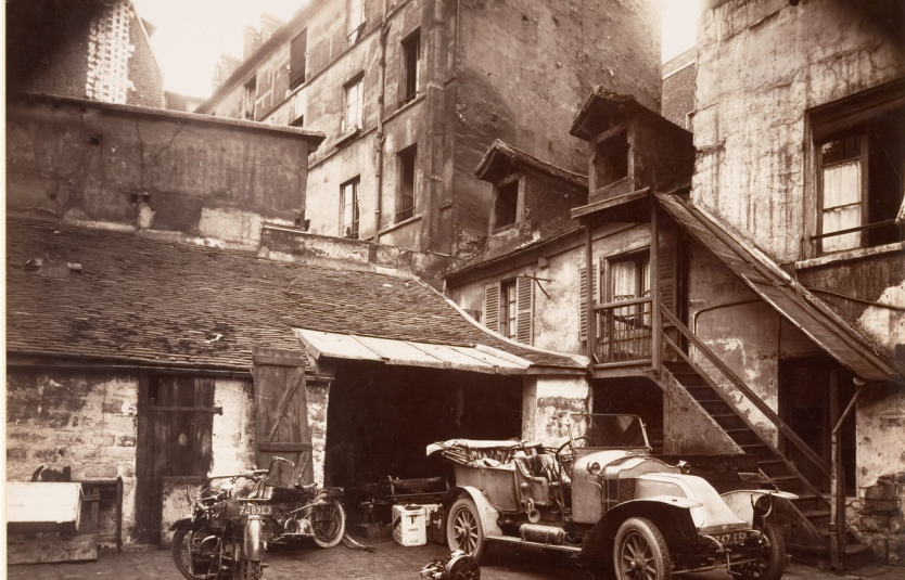
A. The complete courtyard: vehicles, architecture and repair form one spatial system.
